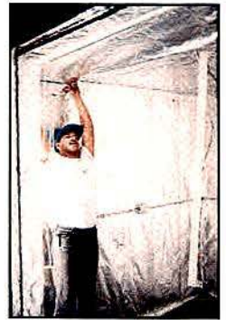
Photos 9-12. John Espinoza (on the left in the first two photos) and Irving Johnson cover the exposed ceiling with spray adhesive and then place the foil. The overlapping junctions are stapled and taped to prevent RF leakage.
