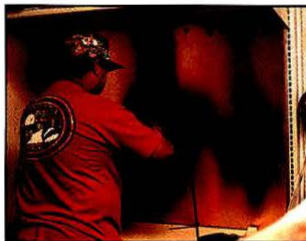
Raymond, my co-worker, cuts the aperture for the ac power lines.
