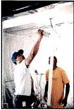
Photos 9-12. John Espinoza (on the left in the first two photos) and Irving Johnson cover the exposed ceiling with spray adhesive and then place the foil. The overlapping junctions are stapled and taped to prevent RF leakage.
