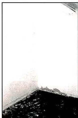
Photo 1. This is the northeast corner of an 8' x 9' x 7' room with a fluorescent light fixture near the center of the ceiling. The walls and ceiling are gypsum-board; the floor is 8-inch concrete.
