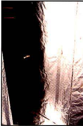
Photo 13. Aluminum foil is stapled directly to the door, folded around it, and then taped to secure the gaps. The door jamb is treated similarly.
